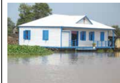
The church in the floating village of Me Chrey was built a year ago
